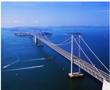
Seto Ohashi Bridge
